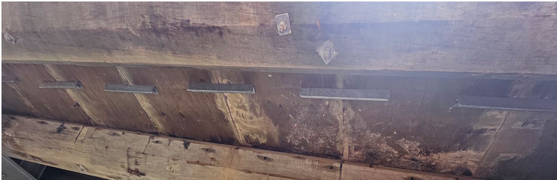
A timber drip strip shall be attached to the outer soffit edge of sheets - refer to Figure 5.2(b).
