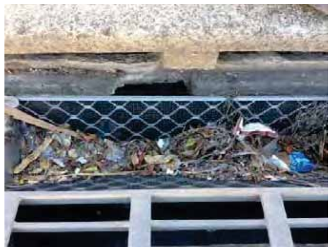
Figure 50a and 50b: Stormwater drain on the southern end of Lamberts Beach could be fitted with a gross pollutant trap to reduce pollutants entering the local marine environment.
